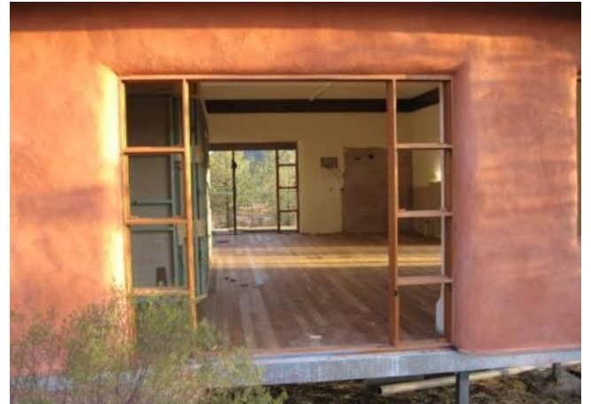
Construction photo of one of the new Villas, now all finished and in operation
